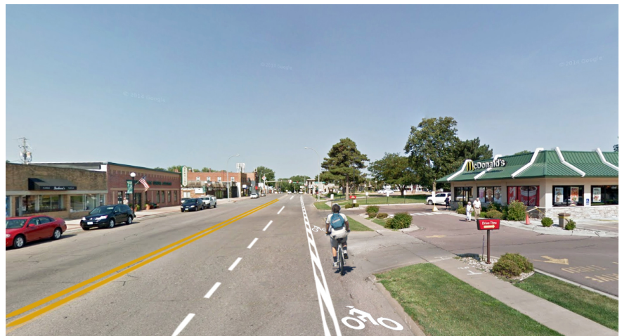
Figure 71. Morningside Ave.: Proposed buffered bike lane.
