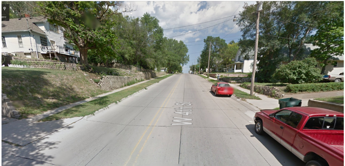
Figure 56. West 4th St.: Existing Condition
