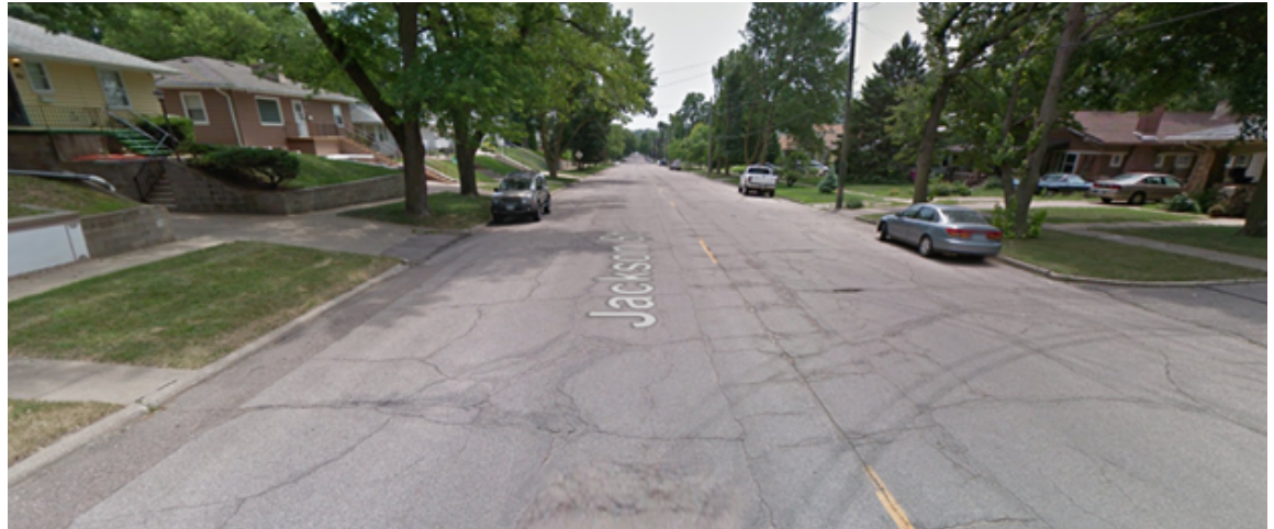
Figure 40. Jackson Street: Existing conditions
