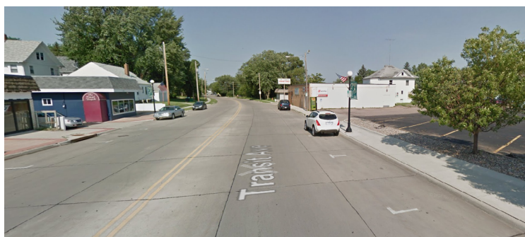
Figure 66. Morningside Ave.: Existing conditions
