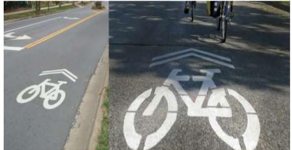
Figure 25: Shared lane marking. Image Source: City of La Crosse Bicycle and Pedestrian Master Plan, 2012.
