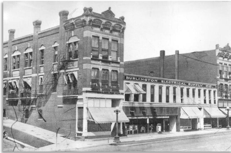
Above: Photograph of the Bookend Buildings as home to Burlington Electrical Supply Co. around 1920.
