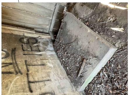
REMOVE CONCRETE PAD
