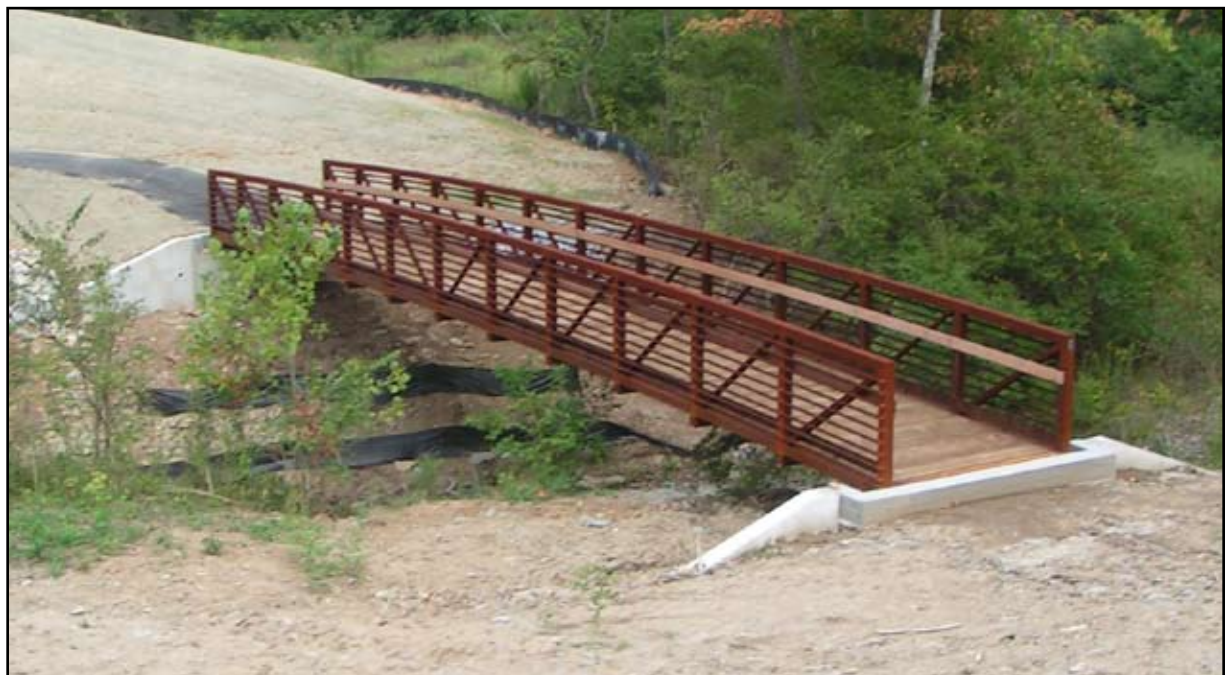
Precast Abutment System installed (Colerain, OH) – Readily available materials and precast pieces means quick installation and overall faster project cycles
