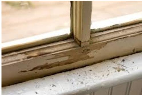
Figure 9.3 Example of lead-based paint inside of a home (Buckfire Law Firm).
