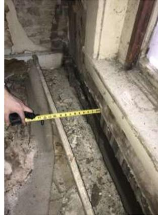
Figure 5. The 4-inch Gap Between the Front Façade and Second Floor Bedroom of Apartment 619.
