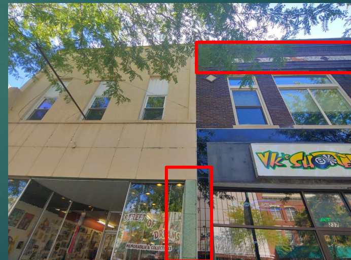
Removal of Stucco Material
