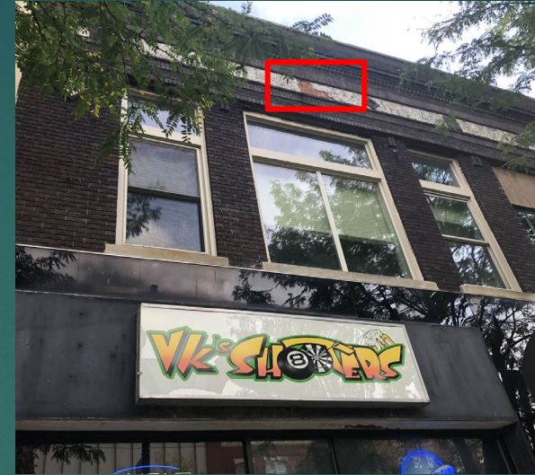
Repointing, Sandblasting & Cleaning
