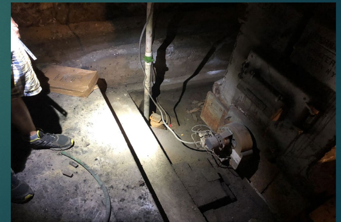
Depressed Boiler Pad
