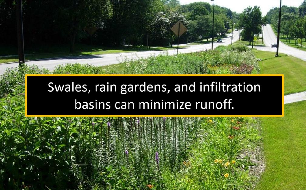
Swales, rain gardens, and infiltration basins can minimize runoff.
