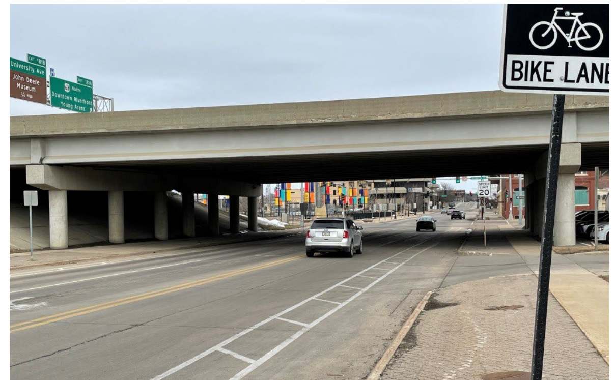
FIGURE 5.3.2 – HIGHWAY 218 UNDERPASS (SOURCE: AUTHORS)
