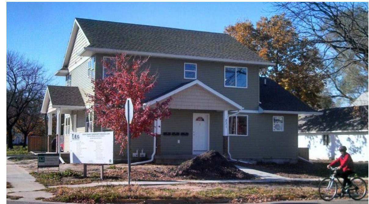
FIGURE 5.1.1 – FOUR-PLEX CONSTRUCTED BY THE SCCHC IN AMES, IA. (SOURCE: STORY COUNTY COMMUNITY HOUSING CORPORATION)
