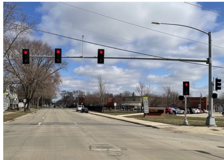
FIGURE 5.3.14 – IRVING ELEMENTARY AT WEST 5TH STREET AND BALTIMORE STREET, FROM THE SIDEWALK. (SOURCE: AUTHORS)
