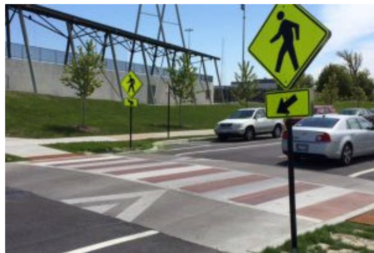
FIGURE 5.3.15 – RAISED CROSSWALK (SOURCE: VISION ZERO FOR YOUTH)
