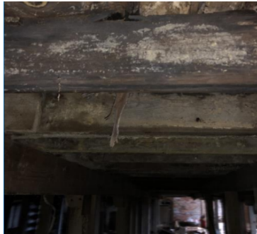
Figure 3: View of main floor framing.
