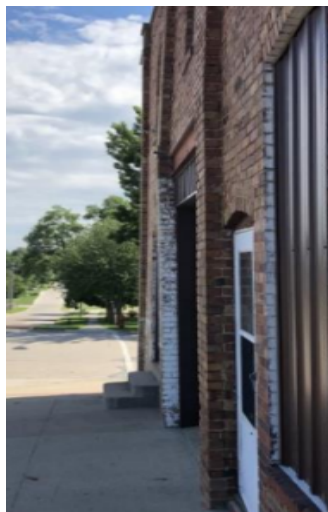
Figure 1: View of bowed facade.
