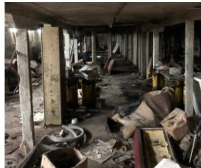
Figure 4: View of floor framing posts.
