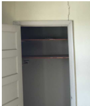
Figure 5: View of Sloped Door Frame
