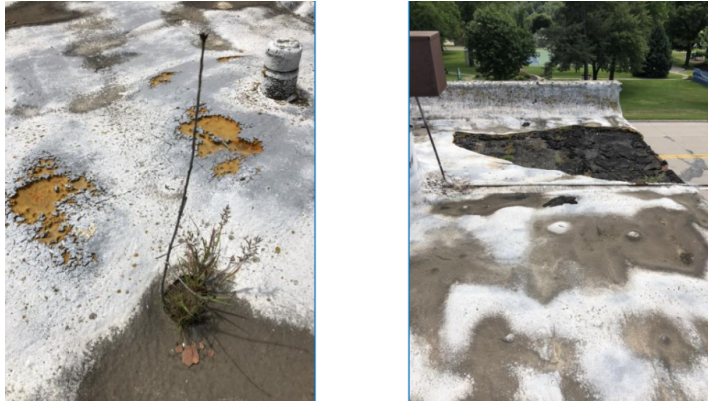
Figure 2: View of exposed insulation and damage on lower roof.
