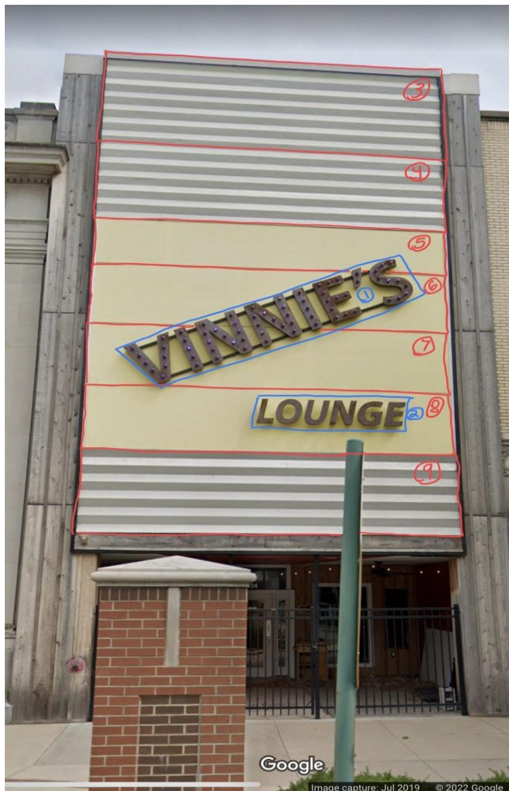
Figure 10: Facade removal steps 1-9.
