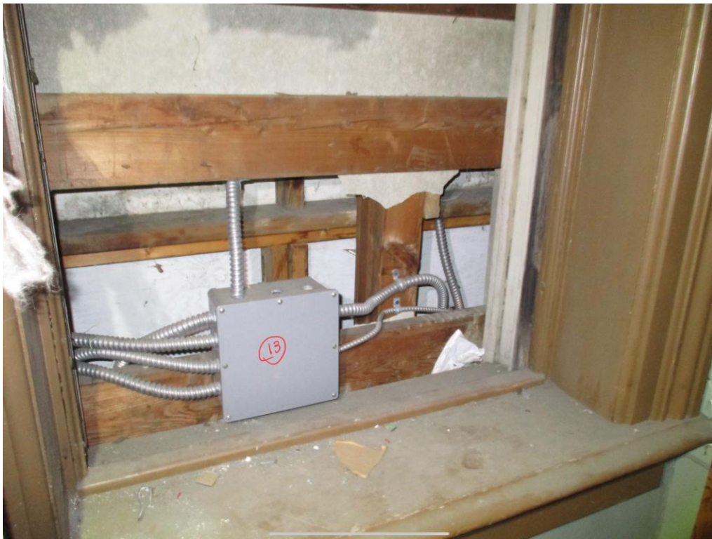
Figure 12: Facade removal step 13
