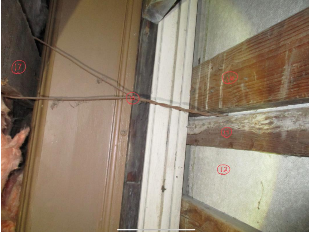
Figure 13: Facade removal steps 12, 14-17.
