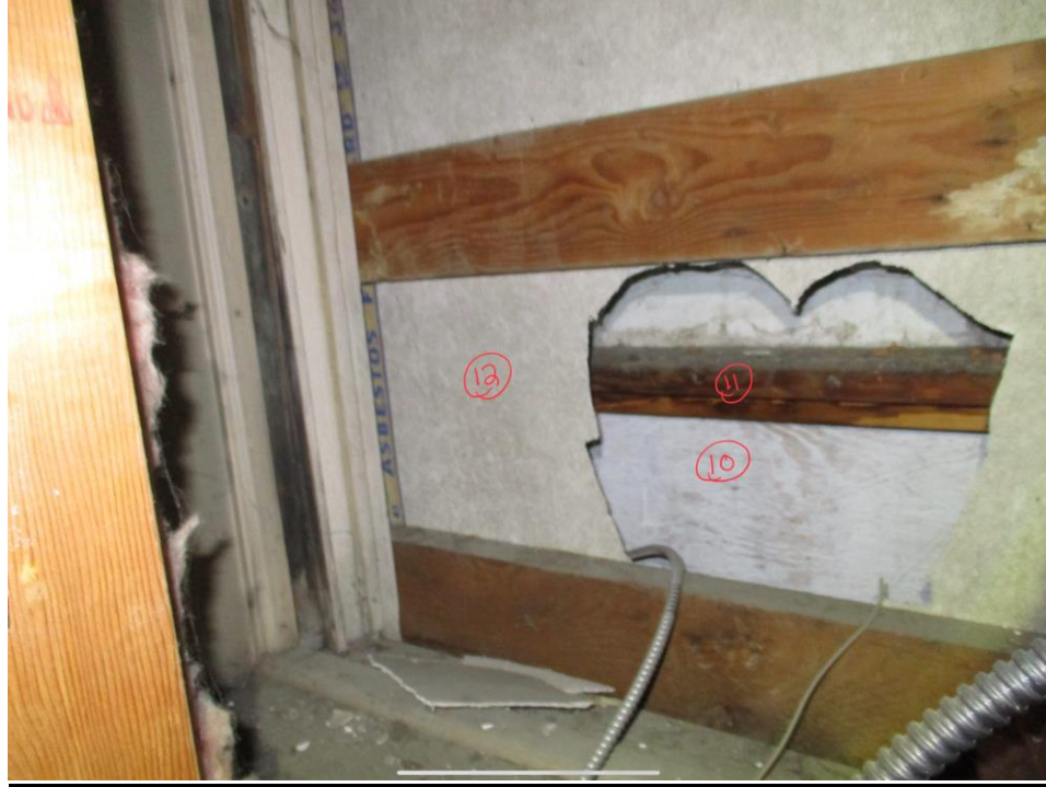
Figure 11: Facade removal steps 11-12.
