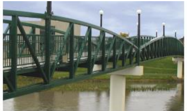
Figure 6.2.5. Weathered steel vs. painted finish.
