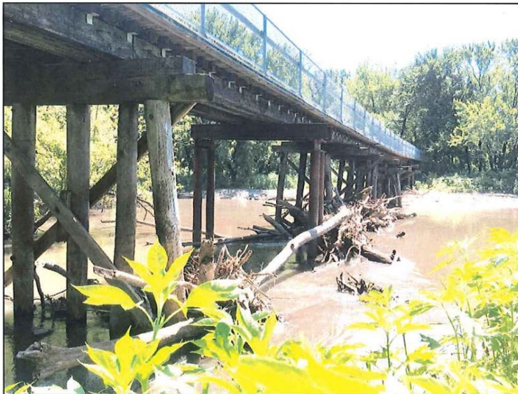
Photo Number: 26 Date: 7/12/2019 Timber pile bent Pier 9 at left, and steel pile bent Pier 8 in channel, looking south
