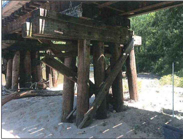
Photo Number: 17 Date: 7/12/2019 Pier 3 looking NE, with two piles missing from north and south bents
