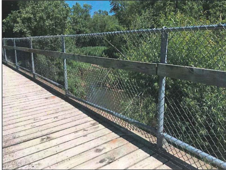
Photo Number: 7 Date: 7/12/2019 Damaged fence member along east side, looking northeast nnn
