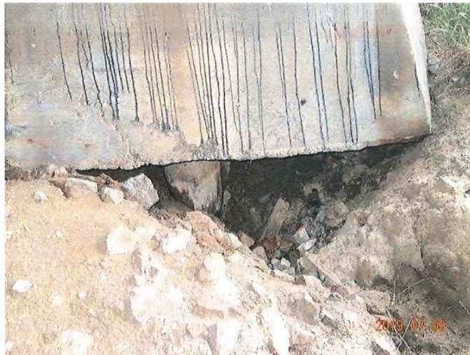
Photo Number: 48 Photo Taken: 07/09/2019 Exposed timber pile at south end of East Abutment cap
