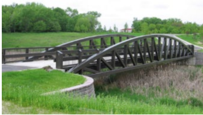
Figure 7: Keystone Truss Bridge
