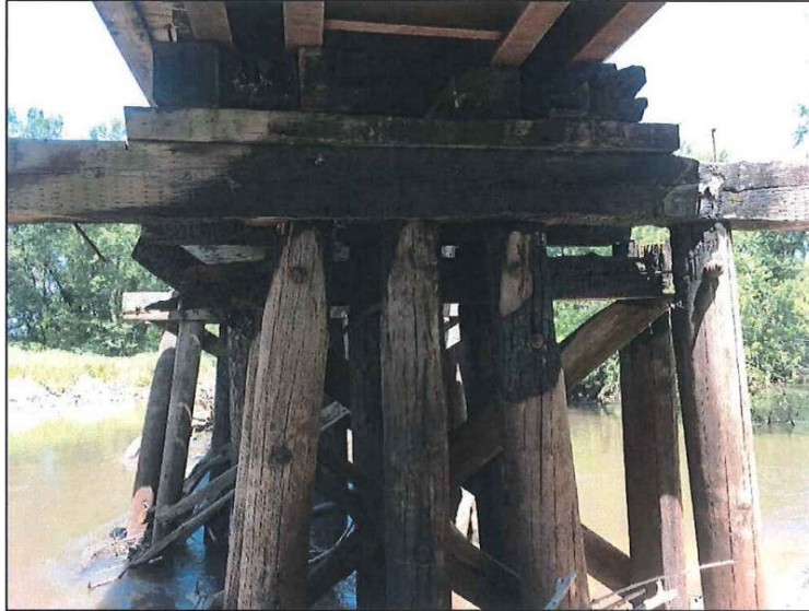
Photo Number: 21 Date: 7/12/2019 Pier 4 looking north showing missing piles at left and fire char at cap
