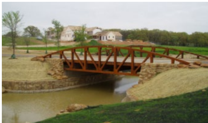
Figure 9: Capstone Truss Bridge
