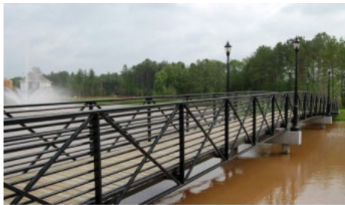
Figure 8: Link Truss Bridge
