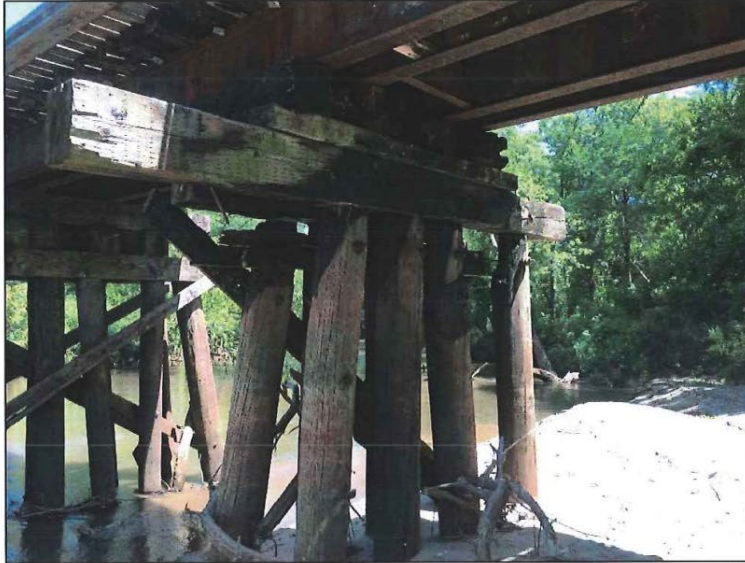
Photo Number: 19 Date: 7/12/2019 Pier 4 looking NE, with two piles missing from the west end of both bents, and fire char on remaining piles and cap
