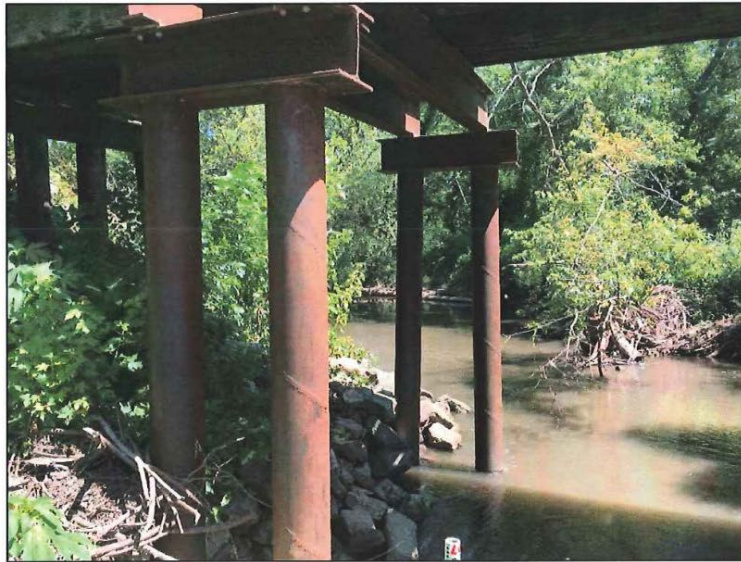
Photo Number: 28 Date: 7/12/2019 Steel pile bent Pier 10, looking NE
