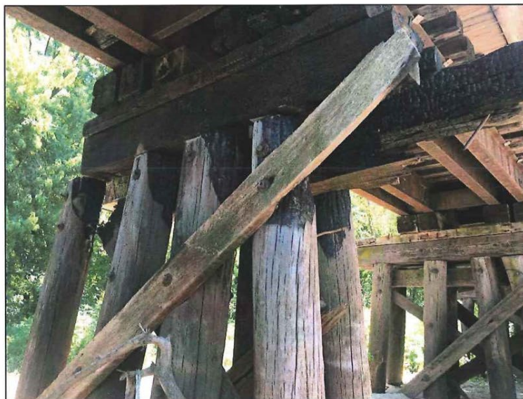
Photo Number: 20 Date: 7/12/2019 Pier 4 looking SE with missing piles at right and severe char on upper piles and cap
