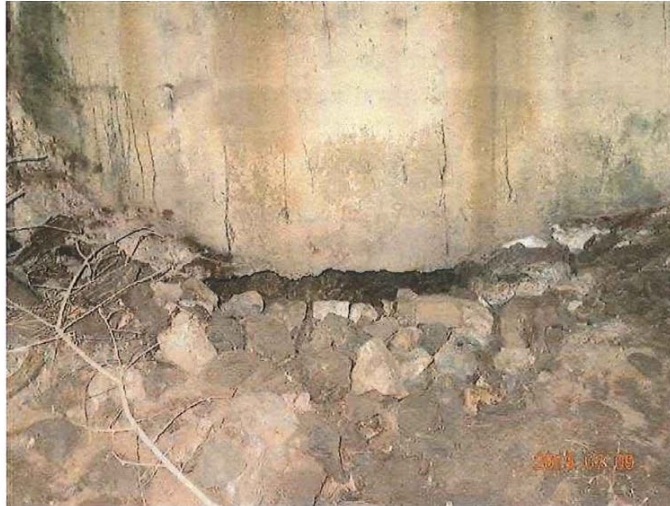
Photo Number: 47 Photo Taken: 07/09/2019 Exposed abutment cap underside at south end of East Abutment
