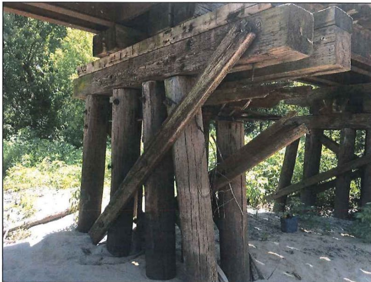
Photo Number: 18 Date: 7/12/2019 Pier 3 looking SE, with two piles missing from west ends of north and south bents
