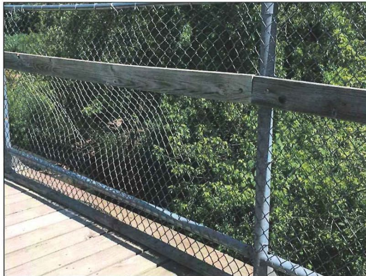
Photo Number: 8 Date: 7/12/2019 Damaged fence along east side, looking northeast
