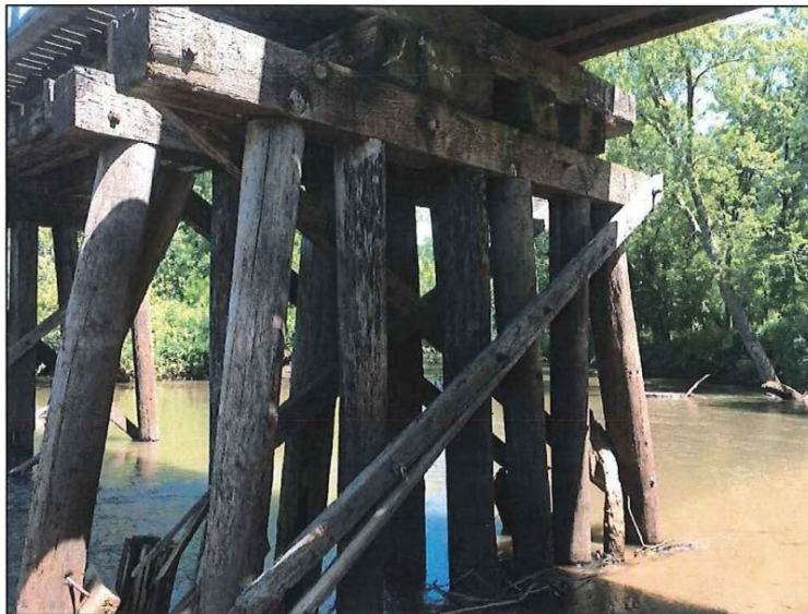
Photo Number: 22 Date: 7/12/2019 Pier 5 looking NW, with pile at far left exhibiting a large split
