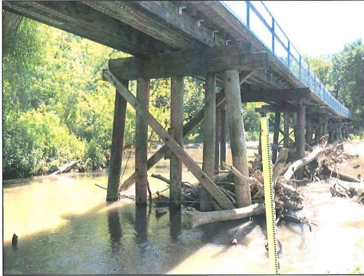
Photo Number: 27 Date: 7/12/2019 Pier 9 looking SE, with large timber debris pile collecting underneath span
