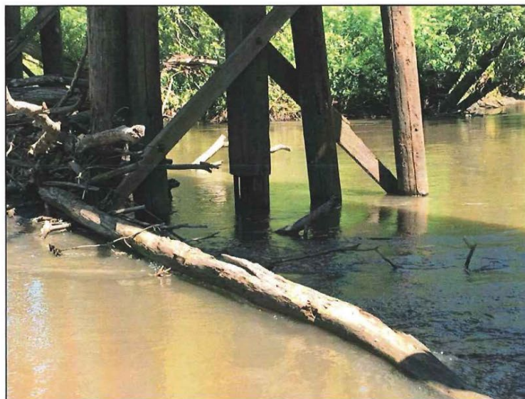
Photo Number: 24 Date: 7/12/2019 Close-up of base of Pier 6, with severe timber decay and partial timber splice visible at waterline
