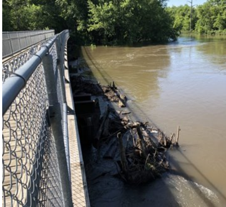
Figure 1: Debris blockage on the northern bridge during flooding
