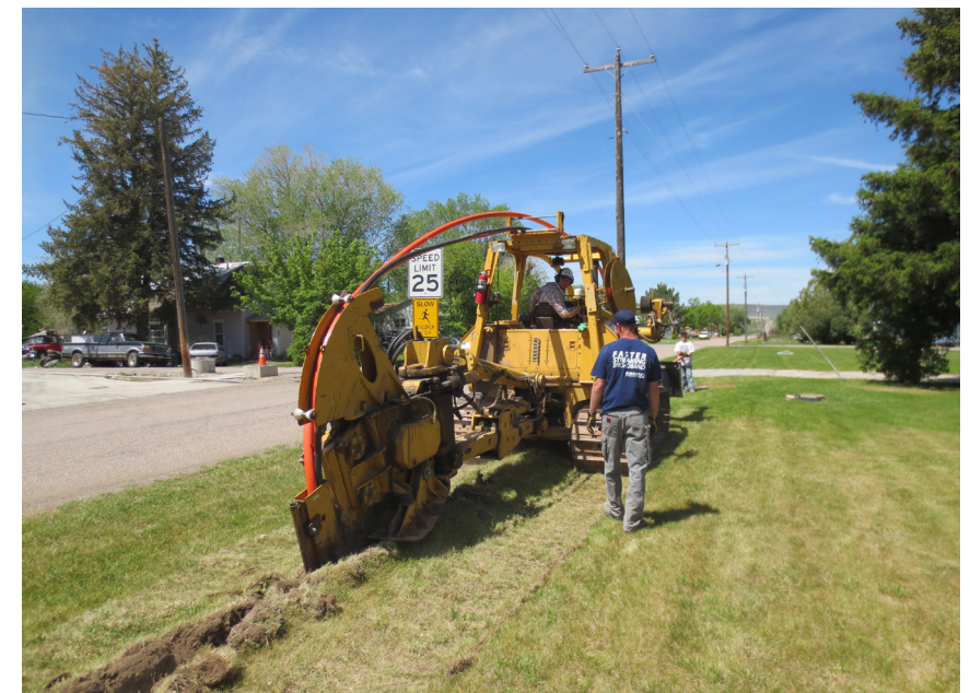
Figure 1.1: REA erecting power lines (Top).
