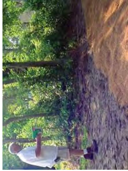
**Figure 14. Stabilize banks daily with lightweight fabric and seeding to reduce the chance of erosion while the wetland develops.**
