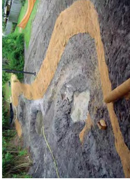
Figure 5. Stabilize the banks each day following excavation of a stormwater wetland.
