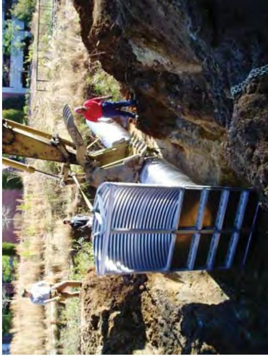
**Figure 9. Installation of a large flashboard riser outlet structure**
