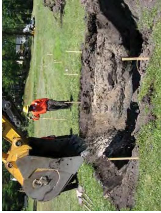
Figure 3. Stake out the wetland perimeter, internal wetland features, and locations of structures prior to excavation. Make sure all existing utilities at the site are located and marked.
