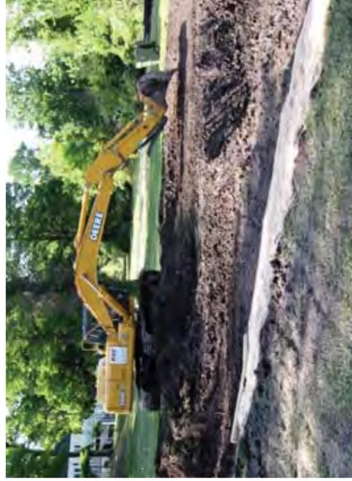
**Figure 12. If possible, keep the excavator out of the wetland and use the bucket teeth for excavation to keep the wetland soil loose for planting. Remember to stockpile topsoil for replacement!**
