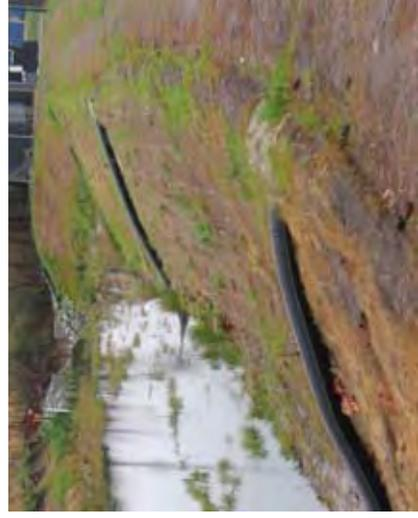
**Figure 15. Two examples of using slope drains for bank stabilization. Surface water generated during larger storms flowing into the wetland is directed into the drains. The drainage reduces erosion that would result from concentrated flow down the banks.**
