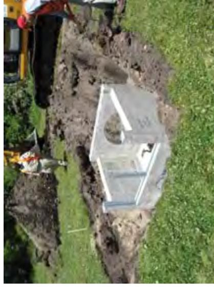
Figure 8. Examples of outlet structures built on-site (top) and prefabricated and delivered to the site (bottom)
