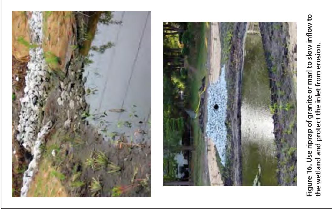
**Figure 16.** Use riprap of granite or marl to slow inflow to the wetland and protect the inlet from erosion.
