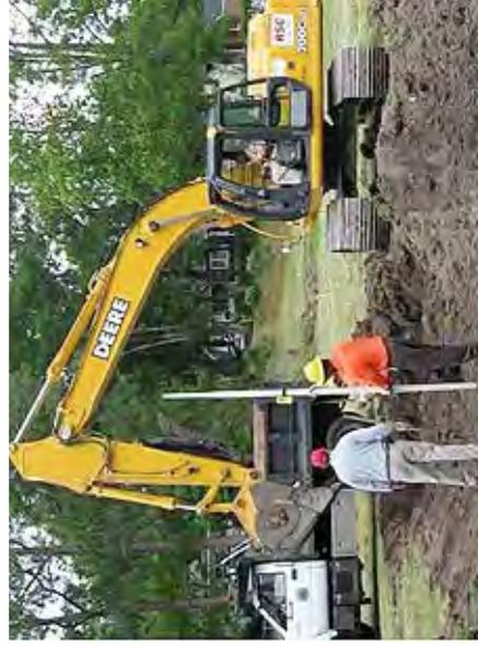
**Figure 11. Keep dump trucks moving for off-site transport of soil (top), and keep the excavator operator updated on correct grade to speed construction (bottom).**
