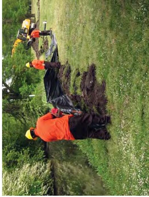
Figure 4. Installation of a silt fence along a stream bank near a new stormwater wetland construction site
