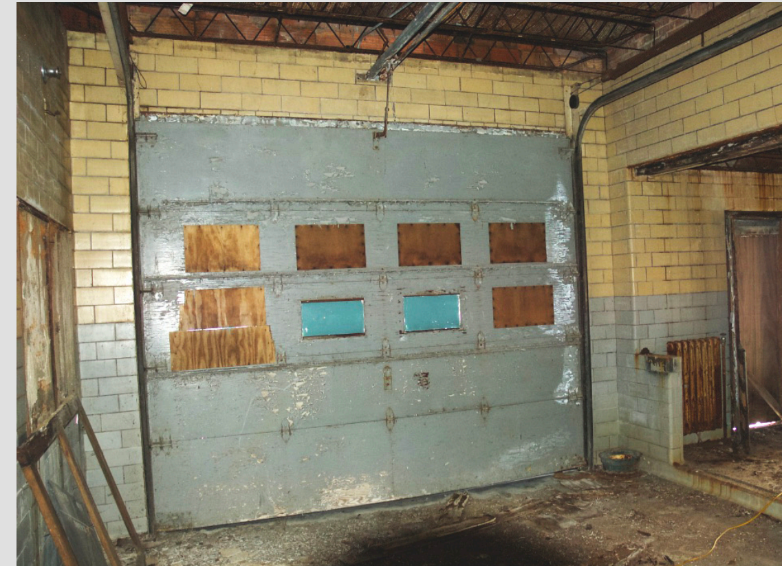
Figure 4: Existing truck bay and overhead door
