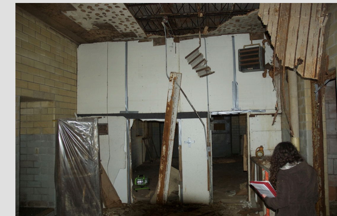
Figure 6: Existing truck bay area
