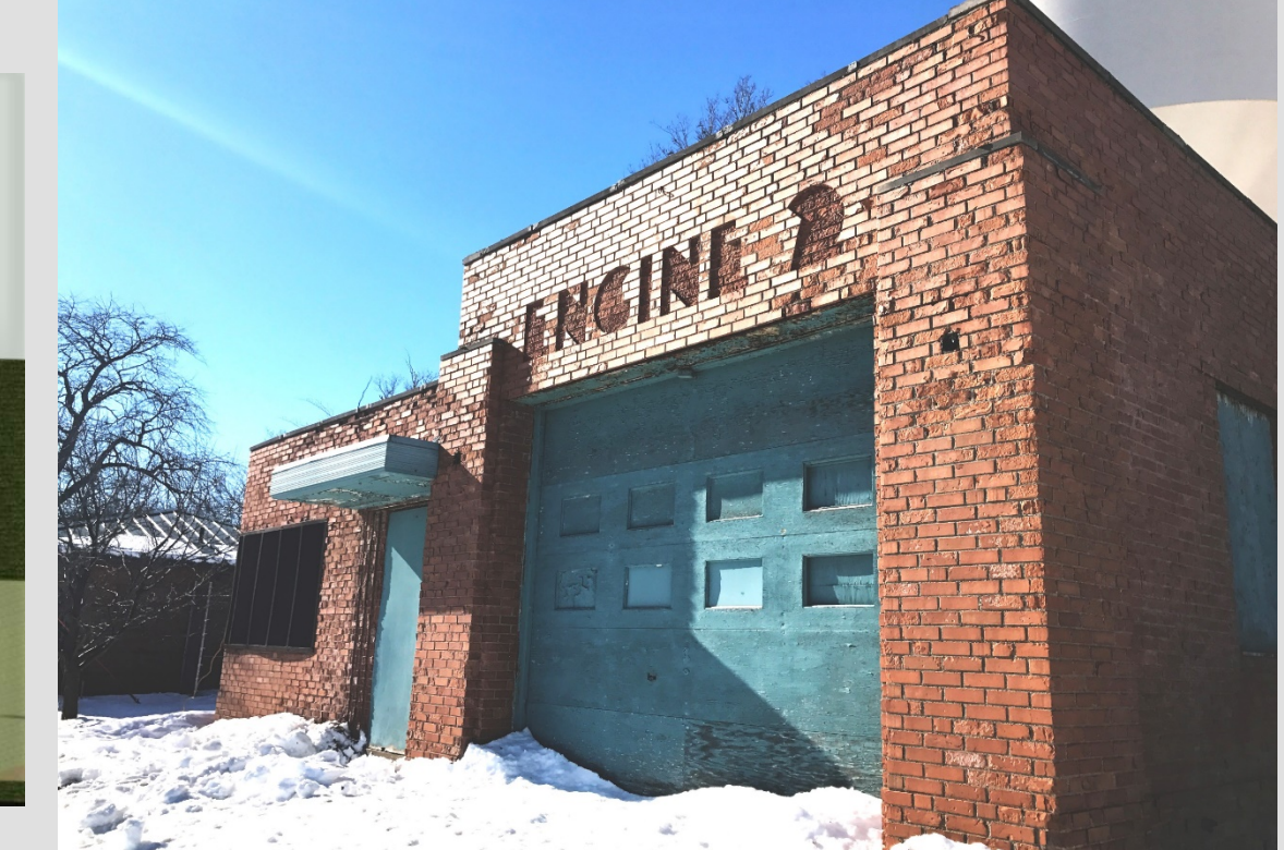
Figure 12: East side current exterior
