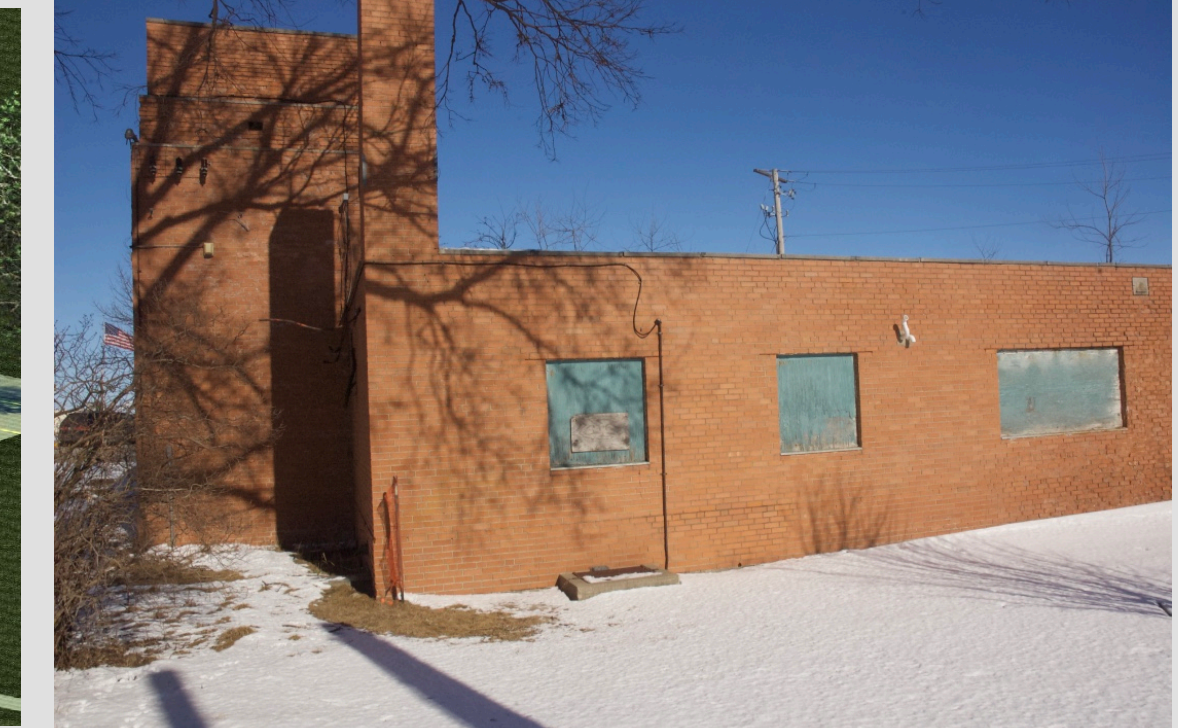
Figure 14: South side current exterior
