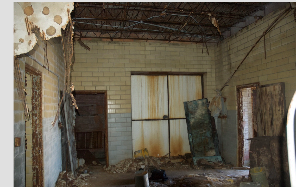
Figure 8: Existing Hose tower and well pump (west wall)
