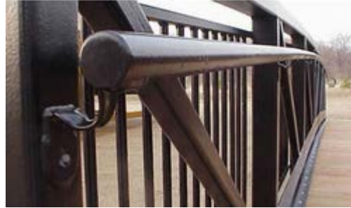
Figure 6.6.3: Vertical picket and pipe handrail.
