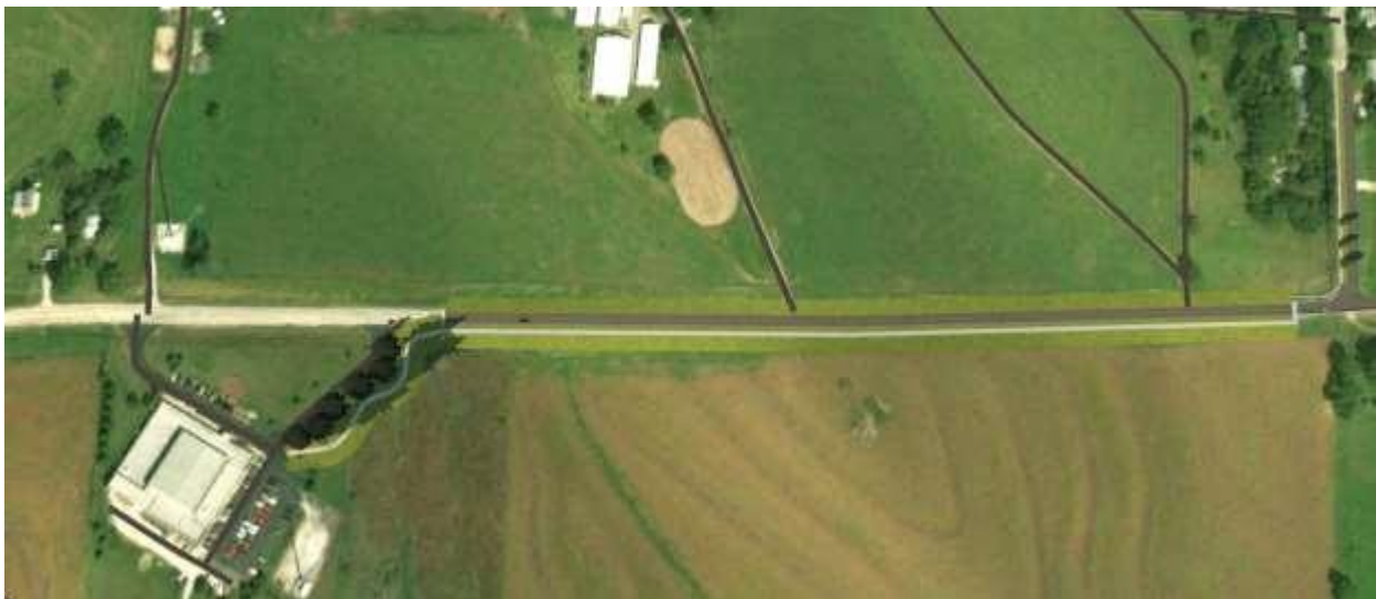
Figure 5.4: shows an aerial shot of the proposed sidewalk
