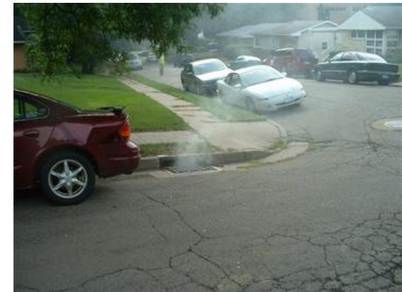
Smoke testing is part of Dubuque's Inflow & Infiltration Program
