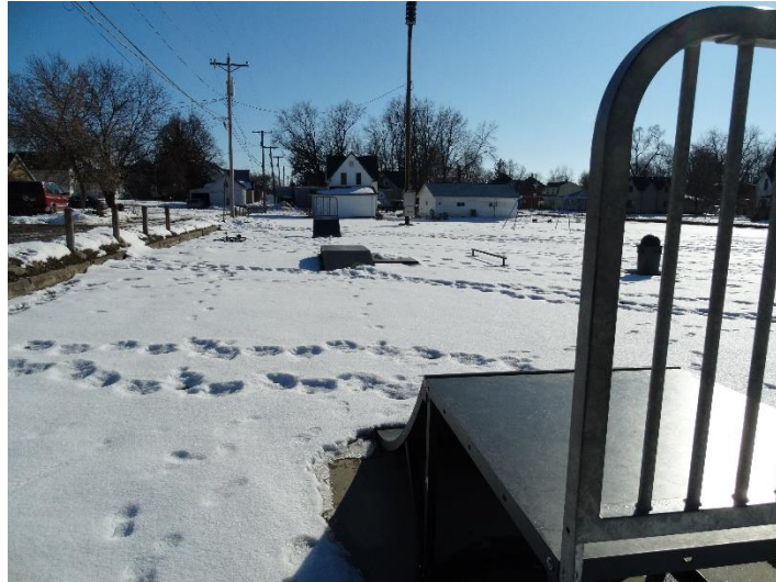
Figure 9.15: Hanging electric lines might be a safety concern especially during a tornado or a storm.
