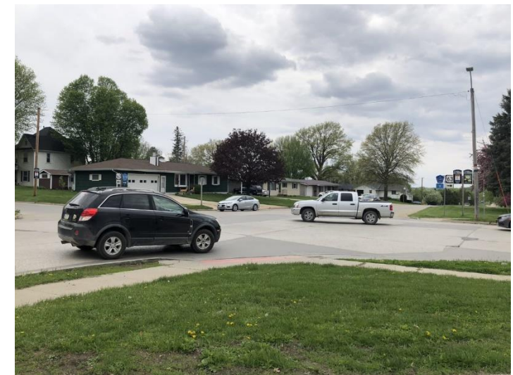
Figure 5.9: Intersection of Harding Street and 13th Street (Hwy 63)
