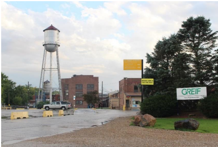
Figure 4.1: Tama Paperboard Mill: an example of industrial uses in Tama
