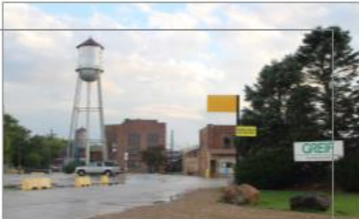
Chapter 6: Infrastructure & Capital Improvement
