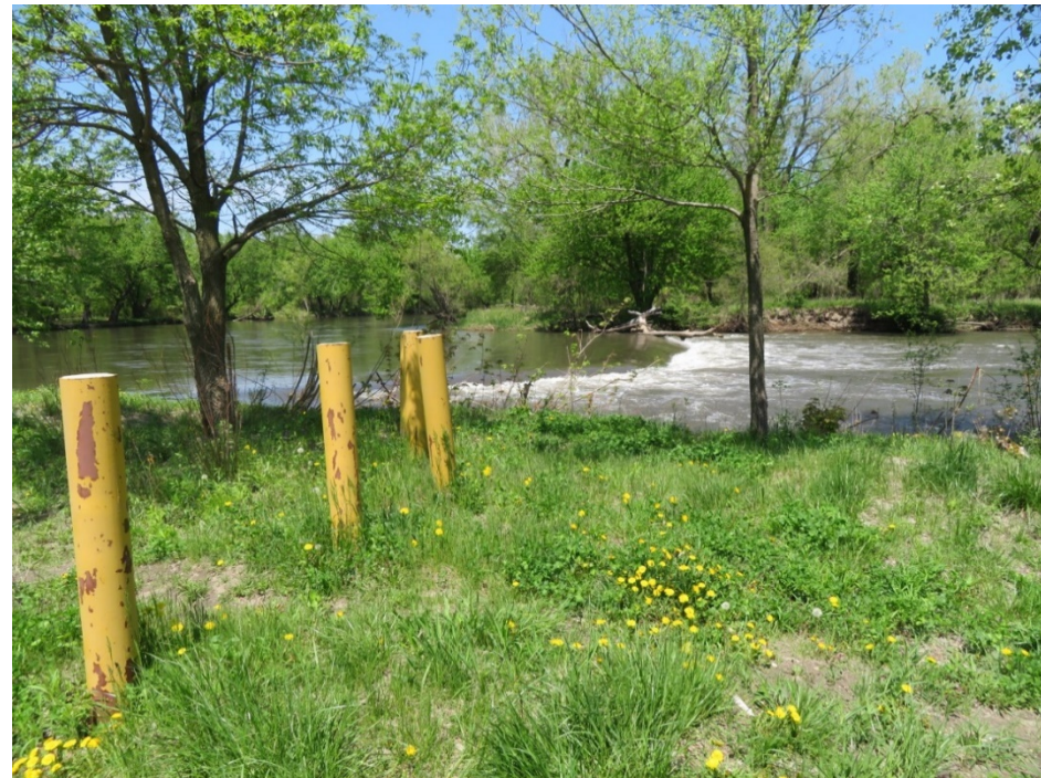
Figure 161 - Water Works Park Low Head Dam – Photo by Lucie Laurian
