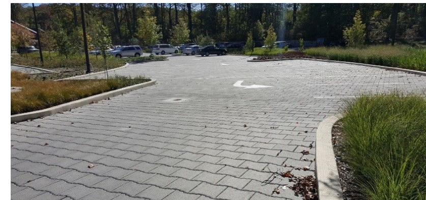
Figure 61 - Permeable Pavement Parking Lot - Brookside Gardens, Montgomery County, MD
