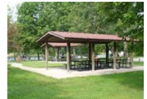
Figure 103 - New Park Shelter
