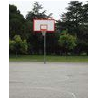
Figure 102 - Resurface Basketball Court
