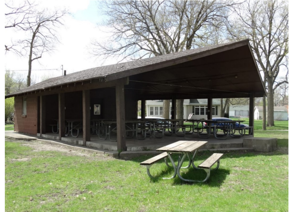
Figure 147 - West Twin Park Shelter
