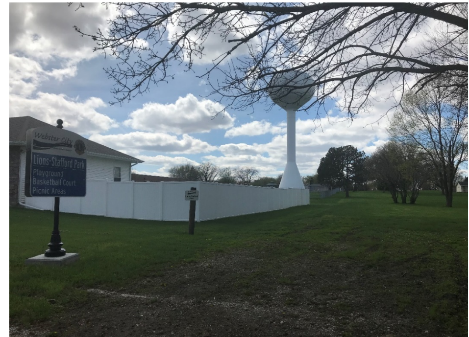
Figure 100 - Signage on east side of Park and Webster City Water Tower
