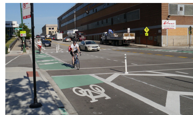
Figure 40 - Intersection Crossing Markings - Chicago, IL
