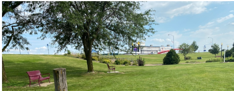
Figure 2: The levee from ground view
