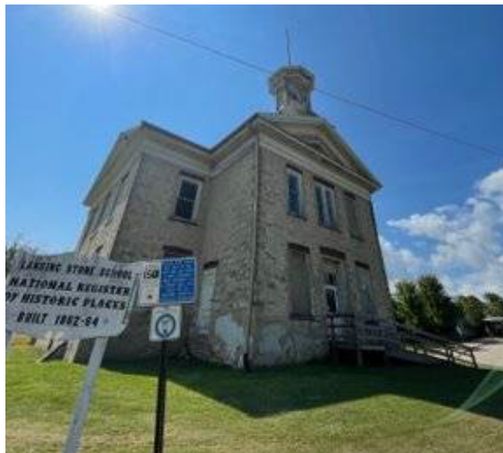
Figure 1: Existing structure pictured during site evaluation.
