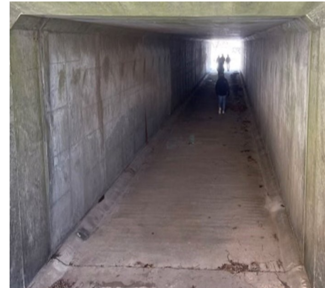
Figure 4: Existing Culvert. Structural modifications are necessary for use in our trail system.
