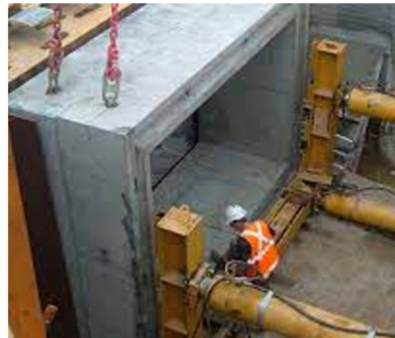
Figure 6: Example Culvert Installation.
