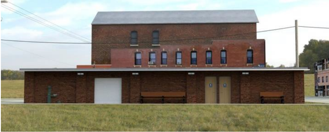
Figure 8B.7. Phase One restroom structure – Front view
