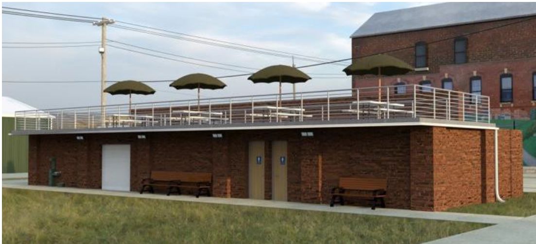
Figure 8B.11. Phase Two restroom structure – Front angled view
