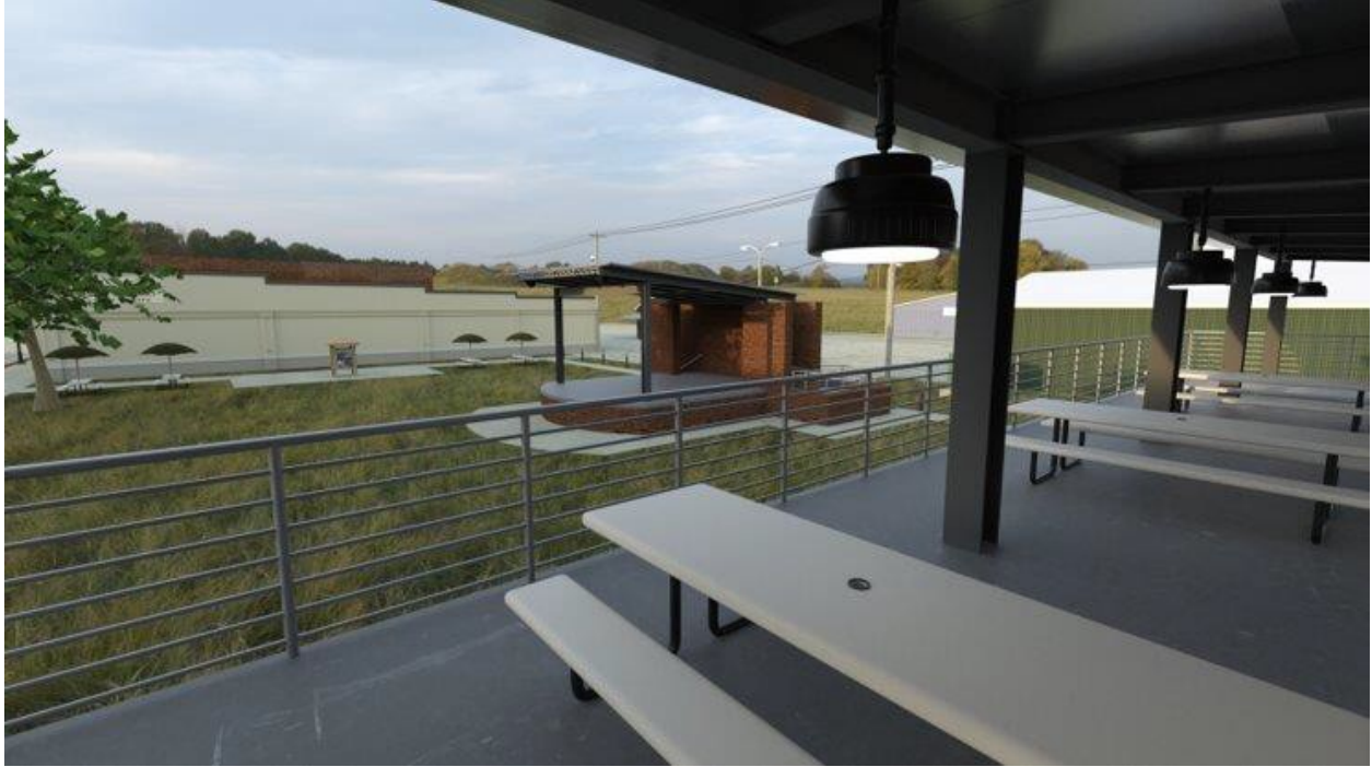
Figure 8B.19. Phase Three restroom structure – Occupiable roof view
