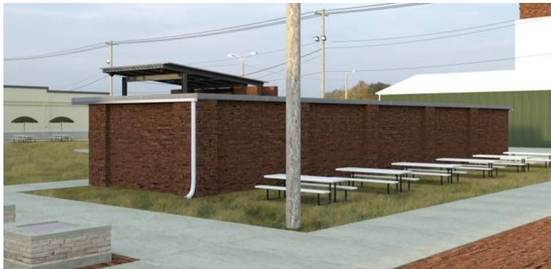
Figure 8B.9. Phase One restroom structure – Back view
