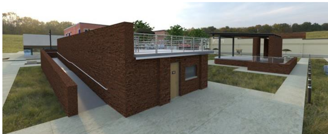
Figure 8B.12. Phase Two restroom structure – Back side view
