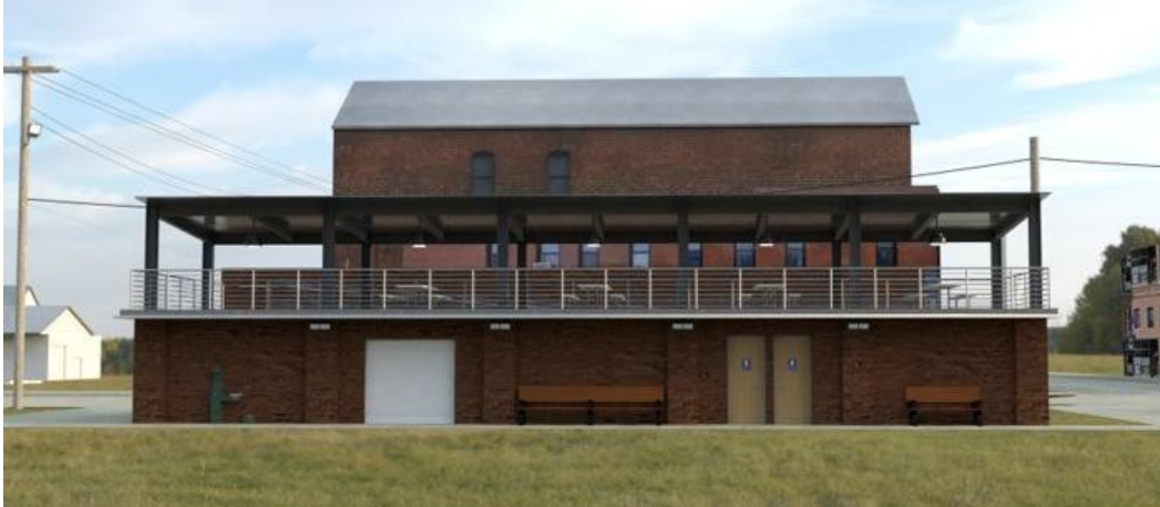
Figure 8B.16. Phase Three restroom structure – Front view
