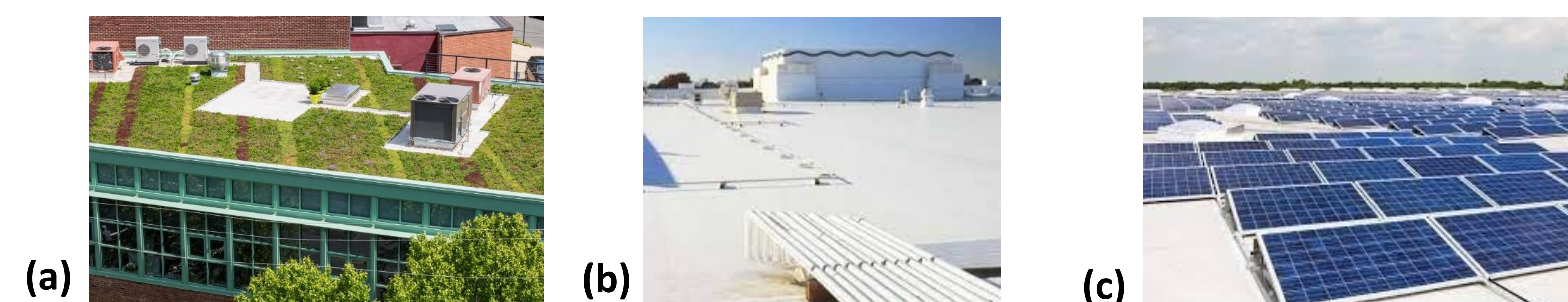
Figure 3. Examples of (a) Green, (b) Cool, and (c) Solar Components of the Roof Design
