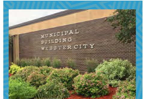
Figure 82: Webster City Municipal Building
