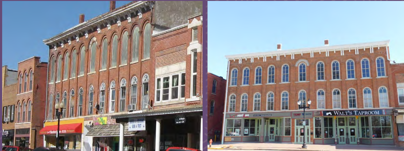
Figure 90: Before and After of The Union Block Building in Mt. Pleasant
