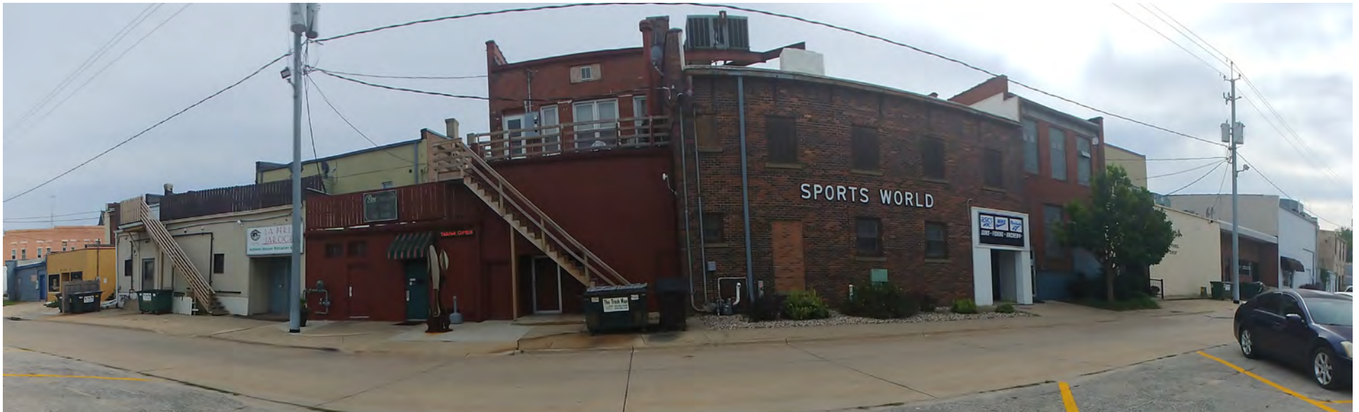
Figure 14: Rear entrances to stores along Second Street
