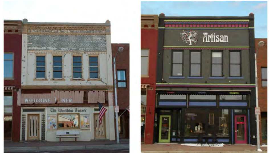
Figure 67: Building rehabilitation in Woodbine, before and after
