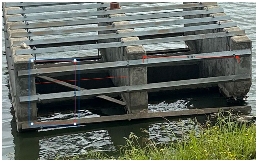
Figure J. 4 Measured outlet structure dimensions
