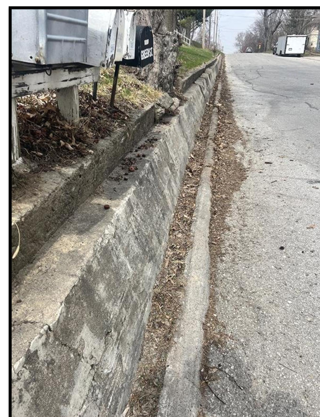
Existing Retaining Wall
