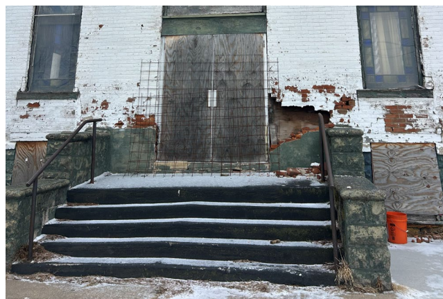
Figure 12. Existing entrance to church
