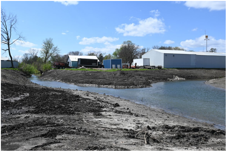
Figure 8.4 Creek Widening Project at the Intersection of Hoover and Wapsi Creeks
