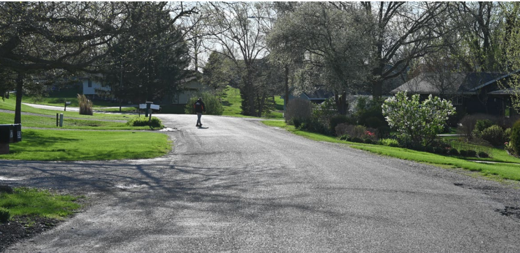
Figure 6.7 Greenview Drive’s Lack of Sidewalks and Road Conditions
