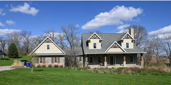
Figure 2.1. A House at the Pheasant Run Development
