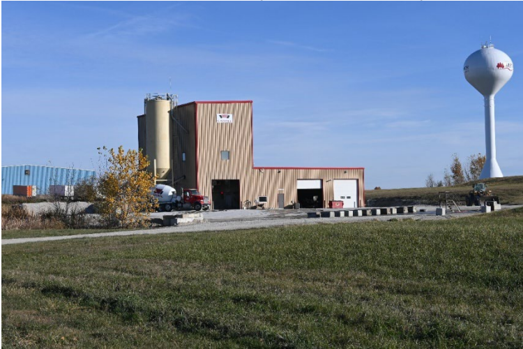
Figure 5.5 Croell: Ready Mix Concrete facility
