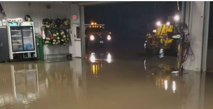
Figure 8.6 West Branch Fire Department Flooding, 2014 Photo Source: WHO Radio, iHeartMedia, 2014.
